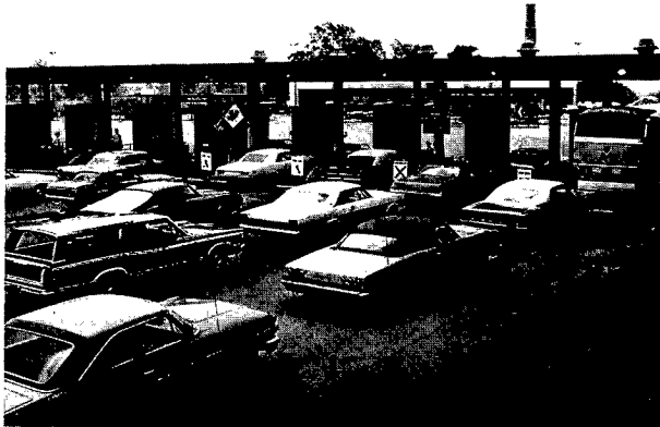
Vehicular inspection at the Peace Bridge, N.Y.
